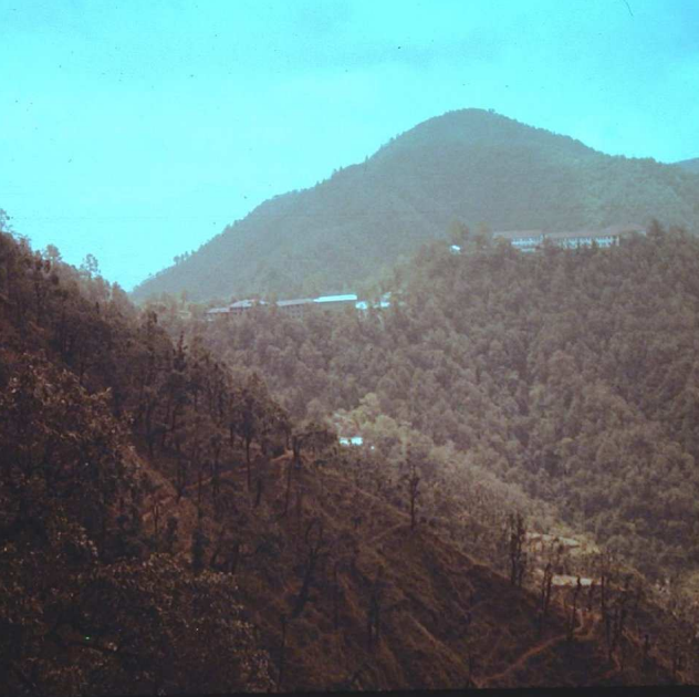
Building on the Hill Side
